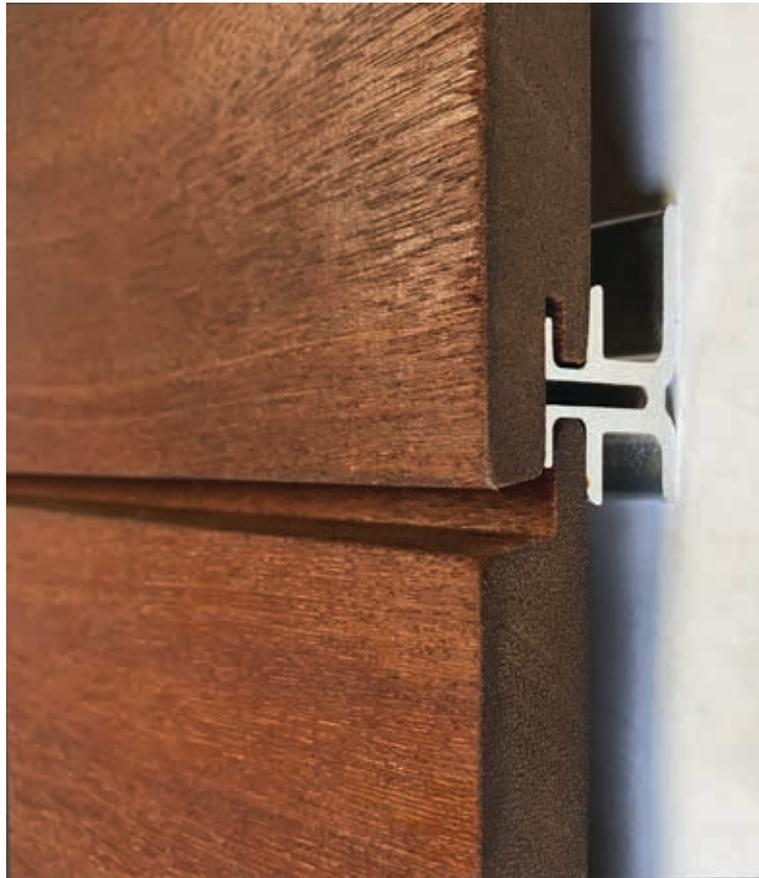
**Resilient clip systems for attaching rainscreen siding accommodate the natural movement of wood as it shrinks and swells with changes in moisture content.**
