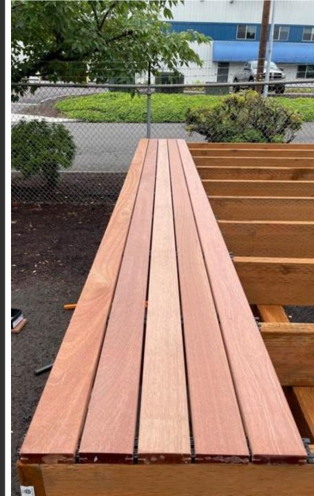
Step 10: If you are using multiple boards to span the length of the deck, ensure that the deck boards butt together properly. The boards should meet in the middle of the joist, with a single clip centered between the two boards. We recommend immediately fastening down the clips at the seems, especially if there is any bow in the boards.
