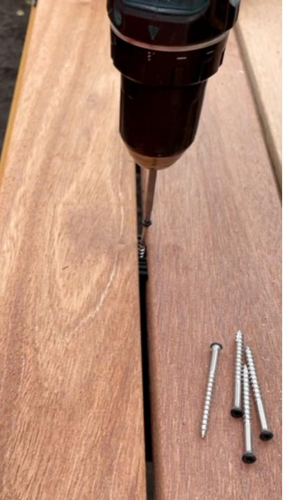
Step 11: Repeat Steps 7-9 until all boards are installed and fully fastened, except your last board.
