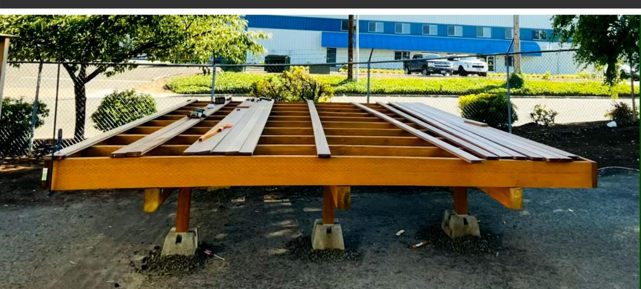
Step 8: If you are using multiple boards to span the length of the deck, ensure that the deck boards butt together properly. The boards should meet in the middle of the joist, with a single clip centered between the two boards. We recommend immediately fastening down the clips at the seems, especially if there is any bow in the boards.
