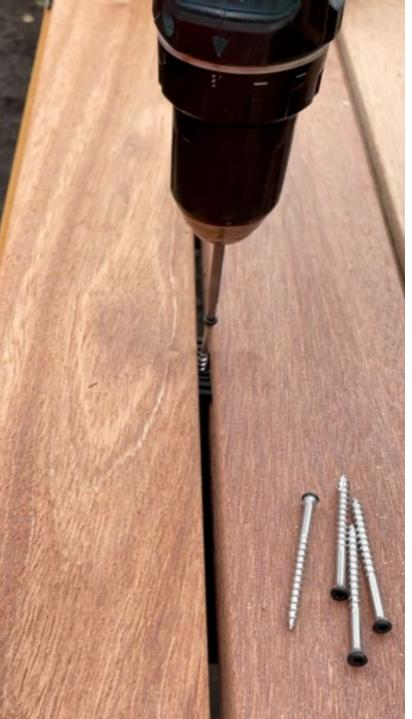
Step 9: Repeat Steps 5-8 until all boards are installed and fully fastened, except your last board.
