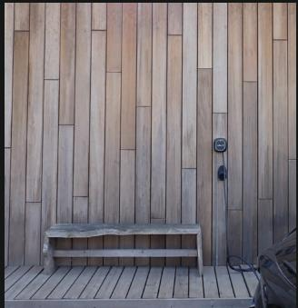
Unfinished S4S siding with hidden fastening clips, and two years exposure.
