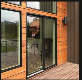
Rainscreen siding installed with hidden fasteners & stained with ExoShield Natural.
