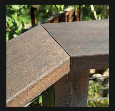
Deck posts and top rail combined with stainless steel cable railing. Decking finished with ExoShield Natural blended with Black Walnut.
